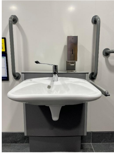
Sink with adjustable height. Press the lever on the right of the sink to move up or down.
